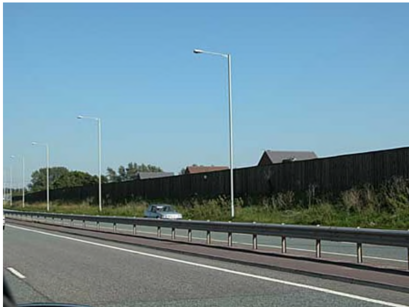
Figure MC6 Example of noise fencing
