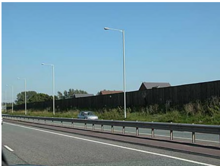
Figure MC1 Example of noise fencing
