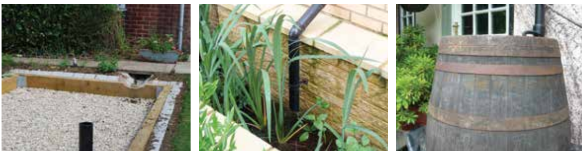
Figure 10.7 On-plot SuDS (courtesy Illman Young, Robert Bray Associates)
