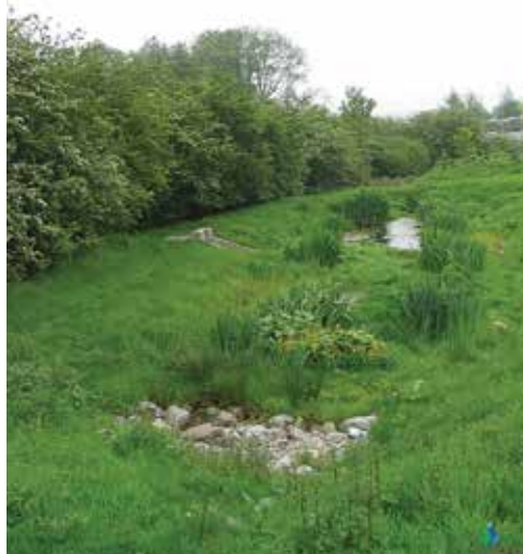
Figure 23.11 Balancing pond with marginal wetland treatment zone, Hopwood Park motorway services, M42, Worcestershire
