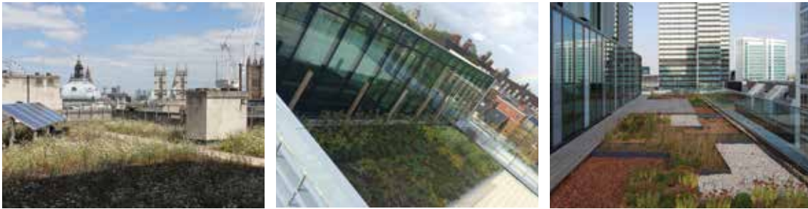
Figure 10.8 Green roofs (courtesy Sky Garden, Arup)
