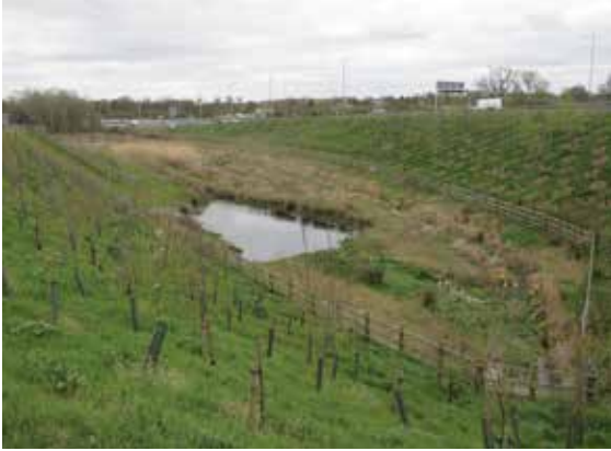
Figure 9.8 Wetland draining a complex traffic island, M4 junction 11, Reading (courtesy EPG Limited)
