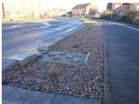
Bottesford retrofit rain gardens (courtesy North Lincolnshire Council)
