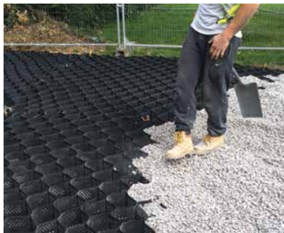
Figure 19.9 Pinning out of cellular confinement system and aggregate infill (courtesy Infra Green Solutions Limited)
