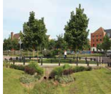
Figure 8.8c Check dams can be combined with road/pedestrian crossings, Upton, Northamptonshire (courtesy EPG Limited)
