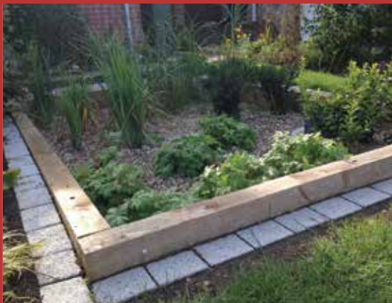
Figure 34.9 A completed rain garden (courtesy Illman Young)
