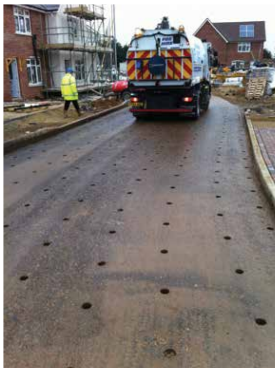
Figure 20.29 Layer of protective DBM over sub-base after coring and before laying concrete block permeable paving (courtesy Peterborough City Council)
