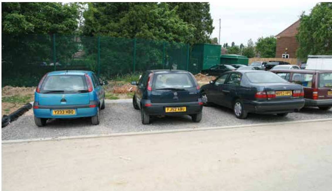
Figure 31.4 Temporary surface over permeable sub-base in parking bays (geotextile and hardcore) (courtesy EPG Limited)
