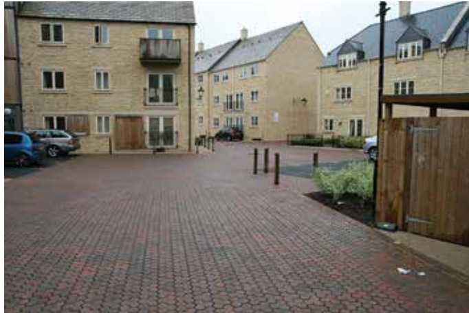
Figure 20.20 Concrete block permeable paving after a 50 mm rainfall event (courtesy EPG Limited)
