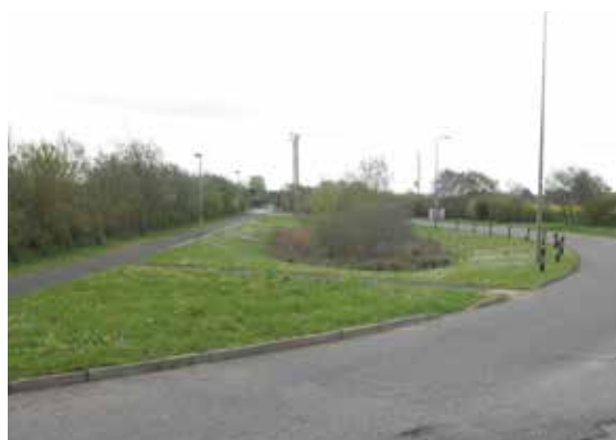
Figure 9.7 Detention basin draining a rural road, Oxfordshire (courtesy EPG Limited)
