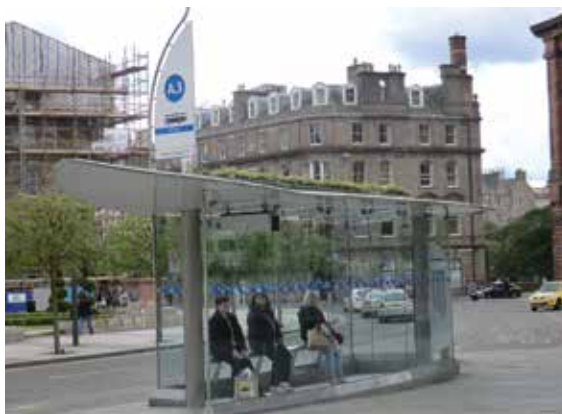
Figure 12.7 Green roof bus stop, Dundee City Centre (courtesy University of Abertay)
