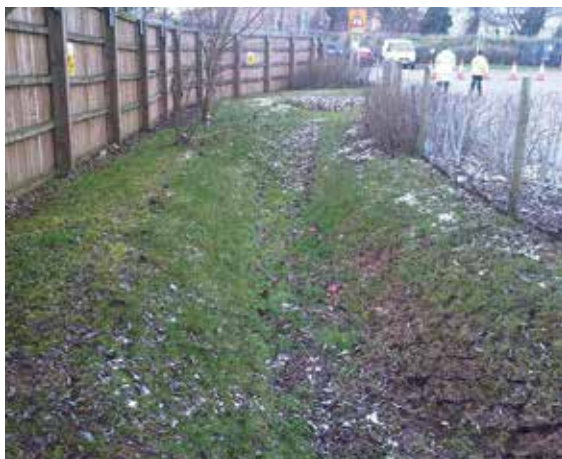
Figure 30.6 Example of topsoil retention on slope using cellular confinement (courtesy EPG Limited)
