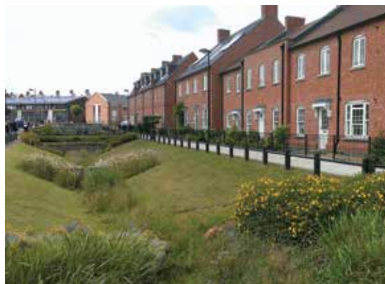
Upton, Northamptonshire (courtesy Peterborough City Council)
