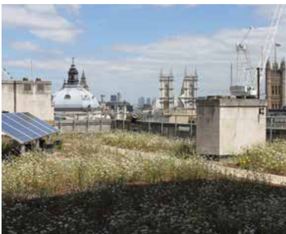
Green roof (courtesy Green Roof Consultancy)
