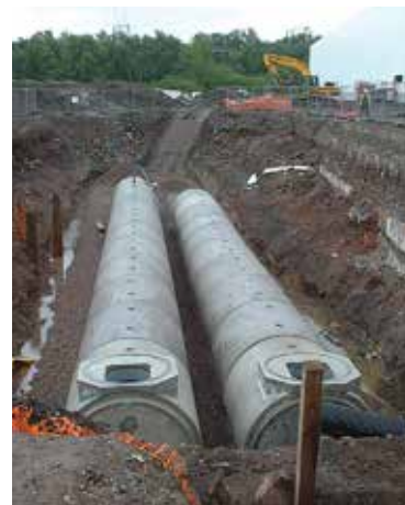
Figure 11.11 Rainwater harvesting storage tanks during construction (courtesy British Precast)
