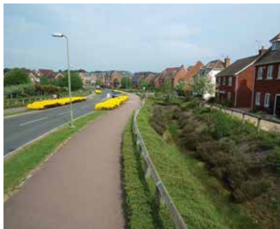
Figure 9.18 Swale set back from road, Elvetham Heath (courtesy Hydro International)
