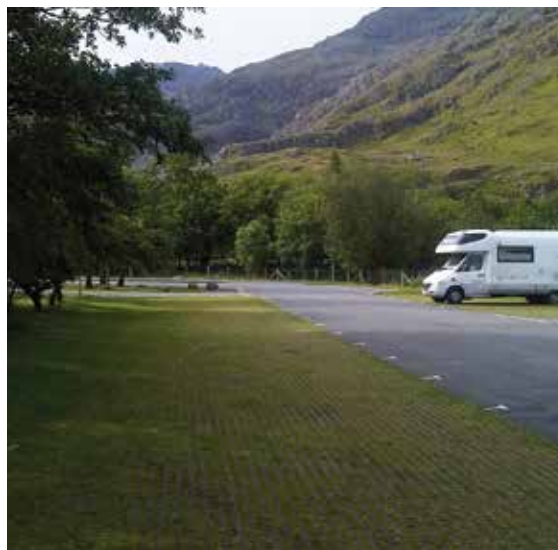
Figure 20.5 Concrete grids in a park and ride overflow car park, Gwynedd (courtesy EPG Limited)
