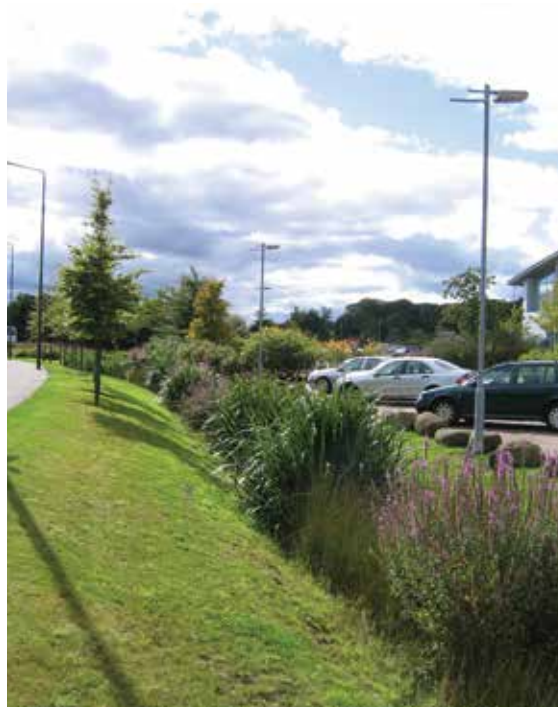
Figure 17.11 Linear wet swale, Junction 4 M8, West Lothian
