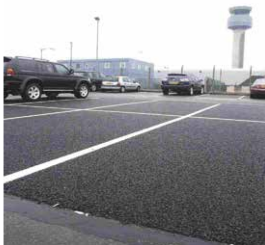
Figure 20.3 Car park at East Midlands Airport with porous asphalt surfacing (courtesy EPG Limited)
