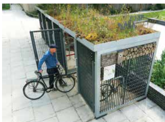
Figure 12.8 Green roof bike shelter at Six Acres Estate, Islington, London (courtesy Green Roof Shelters)
