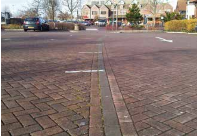
Figure 8.4 Lined permeable pavement constructed over a former landfill site, Portsmouth (courtesy EPG Limited)
