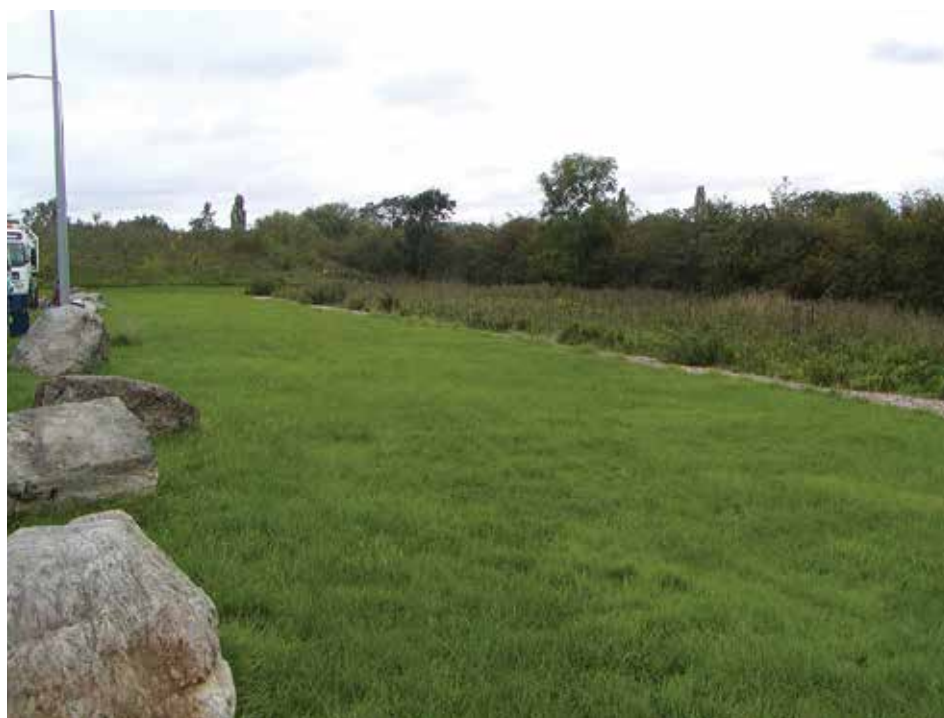
Figure 15.1 Filter strip at motorway services draining to filter drain, Hopwood (courtesy Illman Young)
