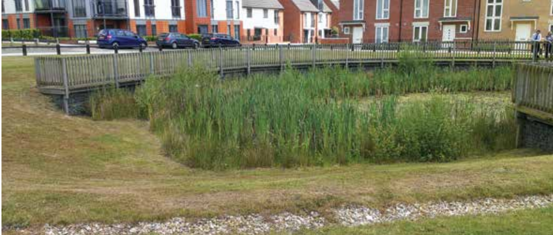
Figure 23.8 Approach to managing risks associated with a steep-sided pond that also adds amenity value, Upton, Northamptonshire (courtesy Peterborough City Council)
