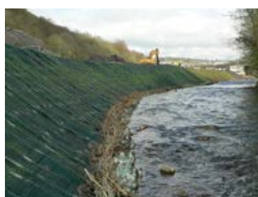
Reinforced mat for grass/planting (courtesy Salix Bioengineering)
