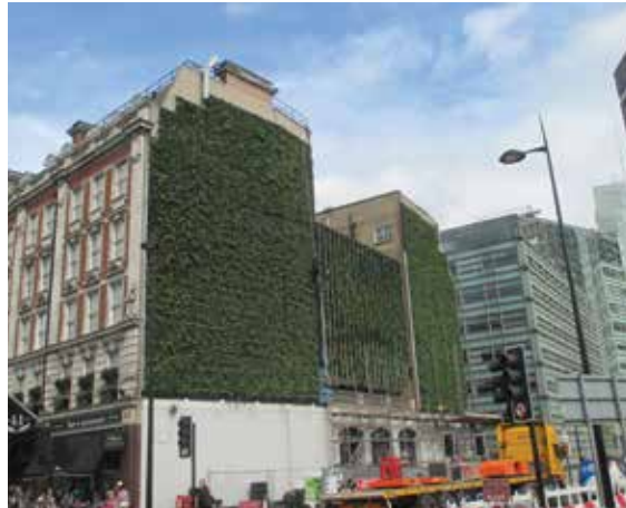
Green wall (courtesy Green Roof Consultancy)
