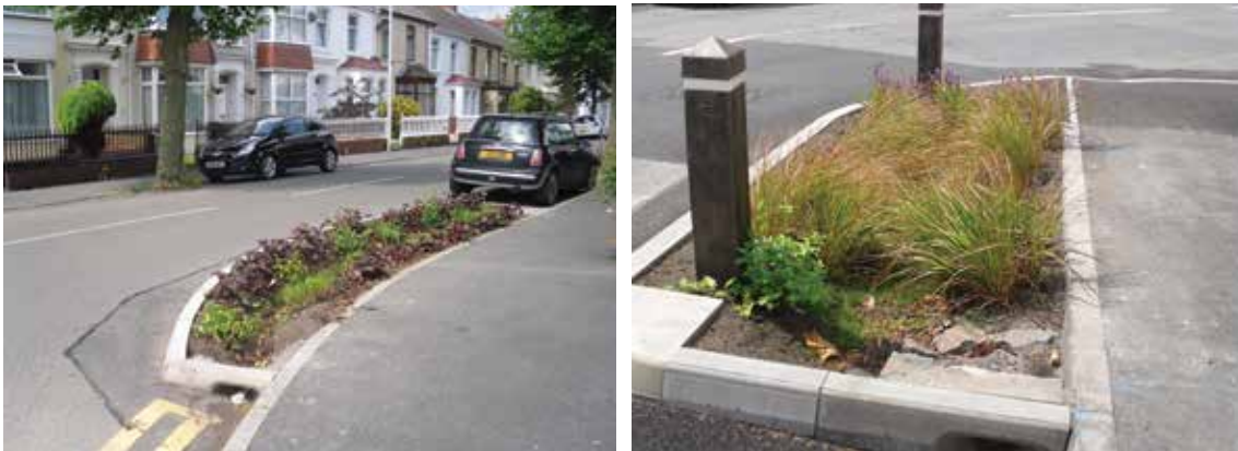
Figure 5.4 Examples of bioretention systems providing traffic calming measures, Llanelli (courtesy Dŵr Cymru Welsh Water)
