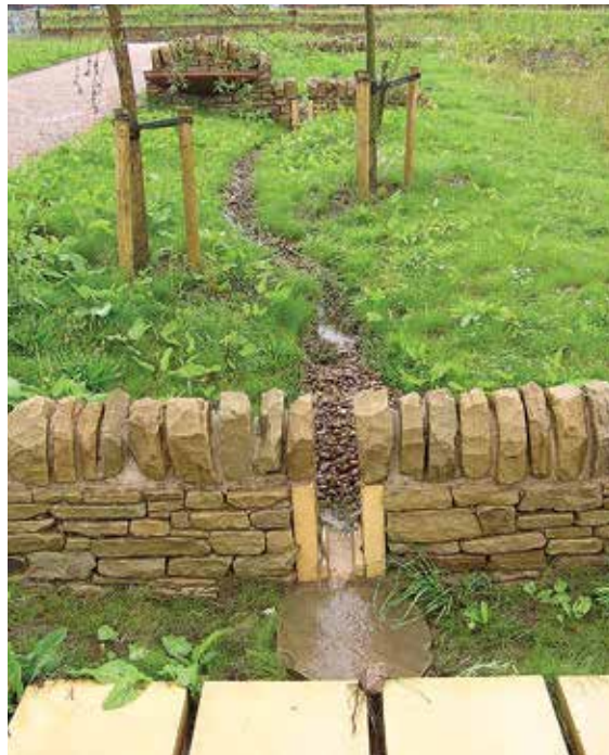
Figure 17.12 Check dam wall using local materials, Sheffield (courtesy Sheffield City Council)
