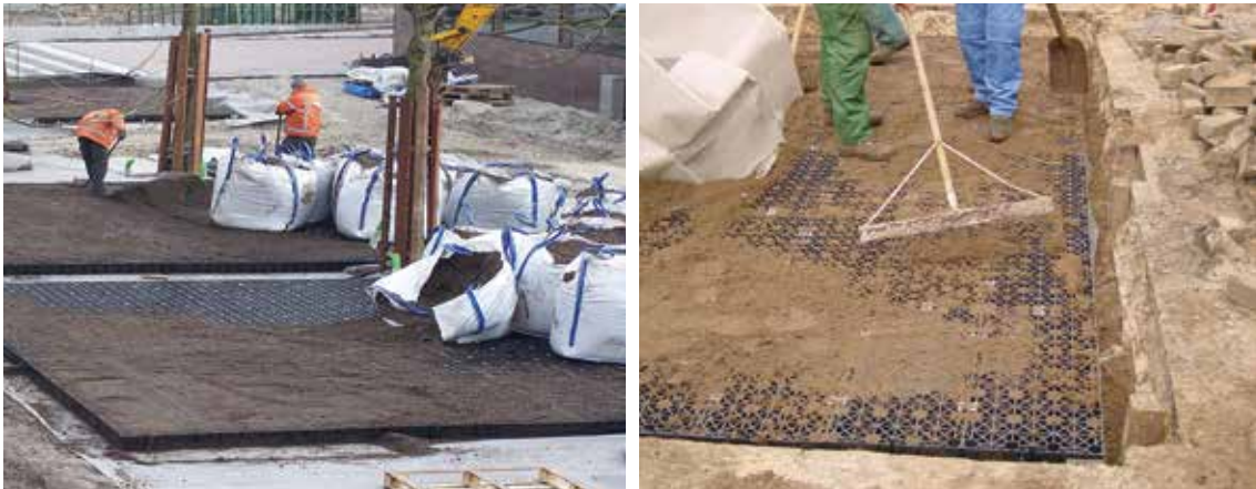
Figure 19.10 Geocellular systems for trees, showing filling of geocellular rafts with structural growing medium (courtesy Permavoid Limited and EPG Limited)
