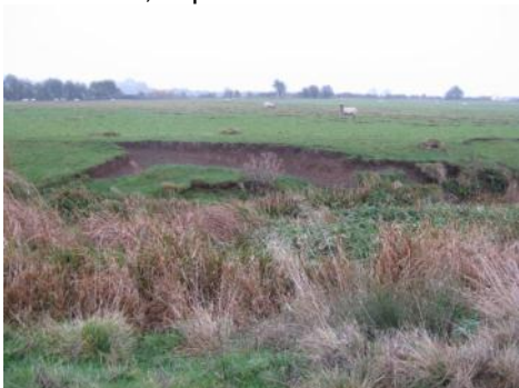
C: Bank collapse
