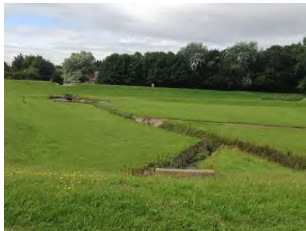
Photograph 3-4: Eastern Catchment 'Winter' Basin
