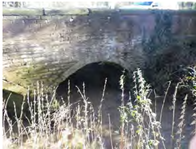
Photograph 4-8: Brick Arch Culvert
